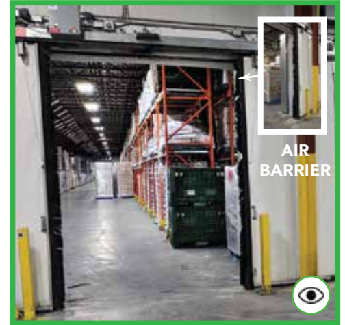
CLEAR LINE OF SIGHT WITH AIR BARRIERS
