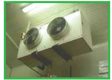
NO FROST BUILD-UP AFTER AIR BARRIER INSTALLATION
