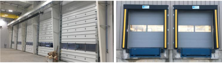
Completed: September 2018 Equipment Provided: (14) Wayne Dalton TS150 Sectional Doors & Liftmaster Model H Operators Nordock CM-66-30K Mechanical Dock Levelers (2) Superseal Model 101 Dock Seals
