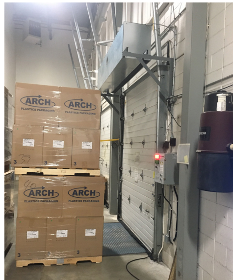
2 OF 3 AIR BARRIERS INSTALLED AT LOCATION #1
