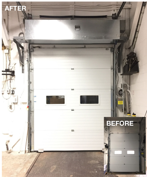
2 OF 3 AIR BARRIERS INSTALLED AT LOCATION #1
