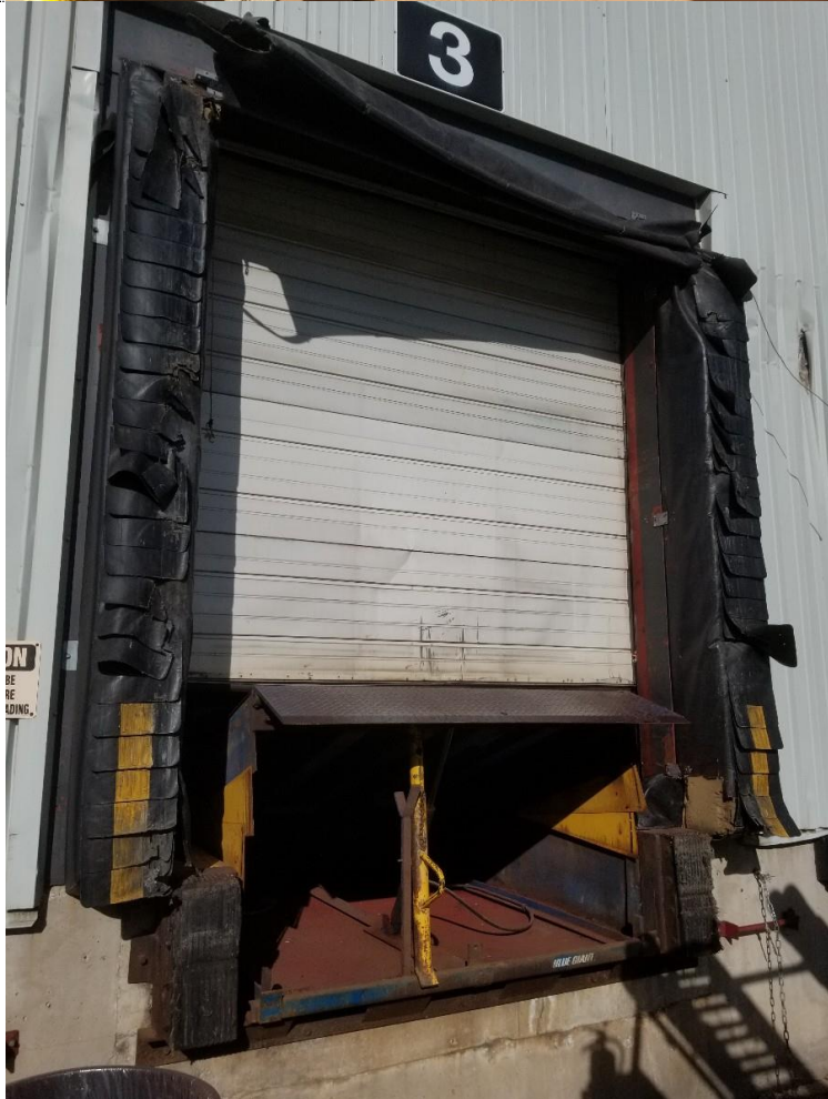
View of worn seal
