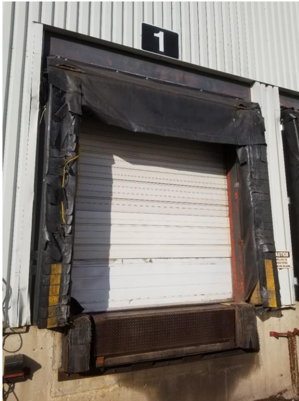
View of worn seal
