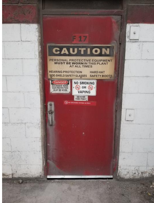
Door F17 – With bottom sweep installed
