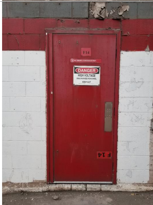
Door F14 – With bottom sweep installed
