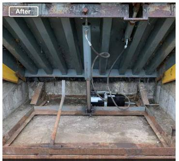
First-time fix with an adjustment on the hydraulic system and clean up one garage bag of debris from the dock pit
